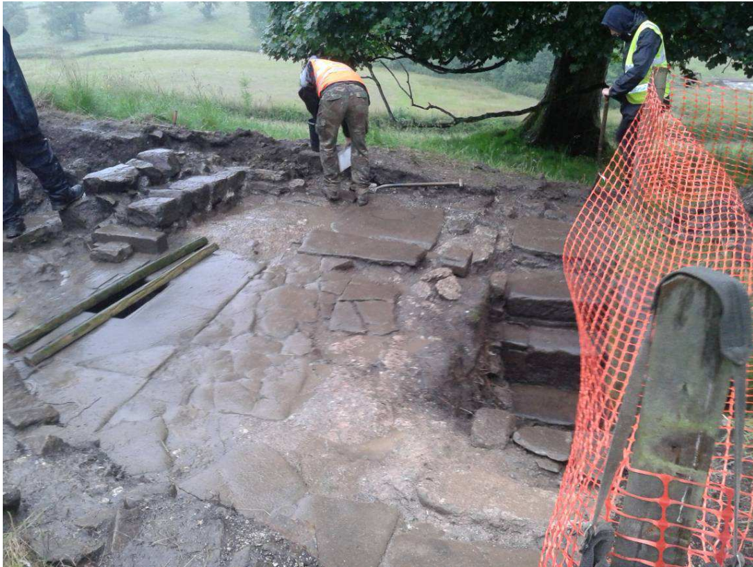
Plate 1: General view of the northern room under excavation, viewed looking north.
