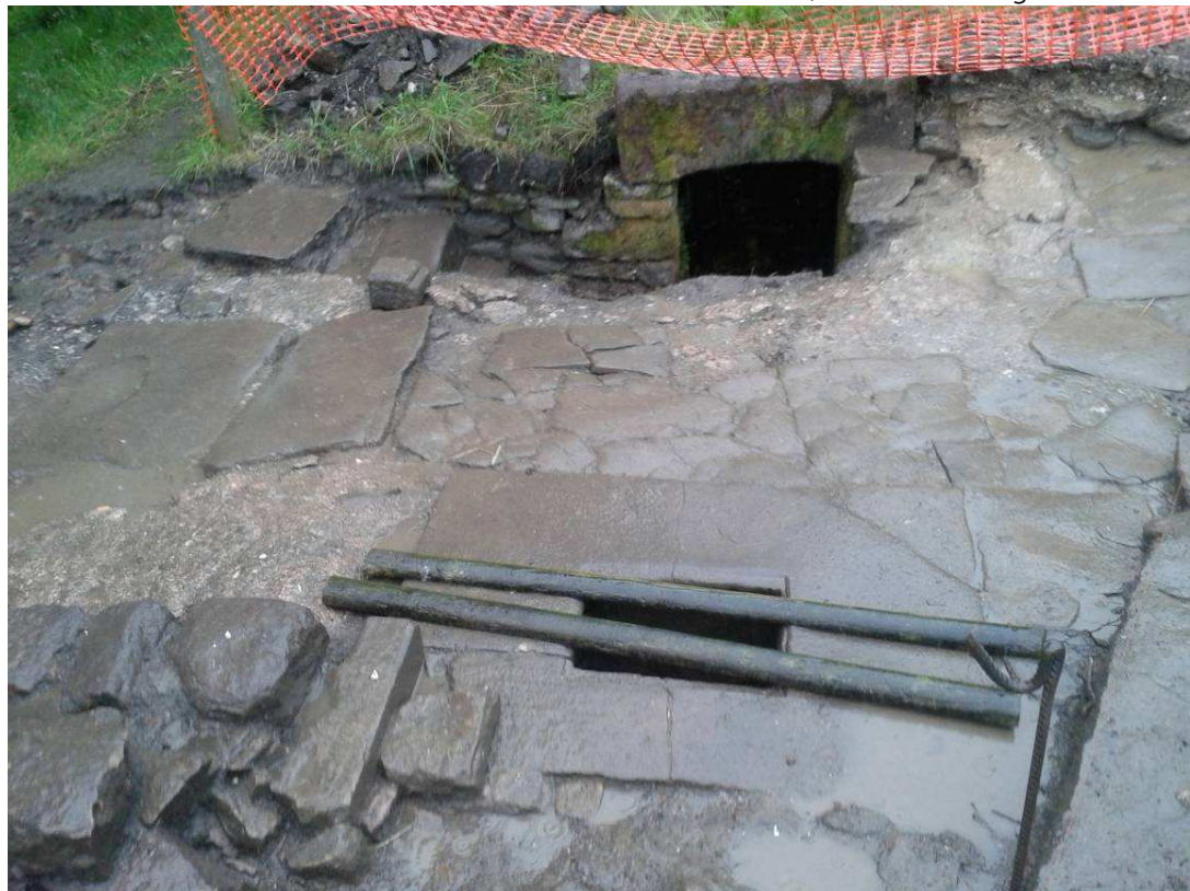
Plate 2: General view of the northern room, viewed looking south-east. Note the later stone flag at the top of the cellar steps and the re-used stone arched lintel leading into the cellar.
