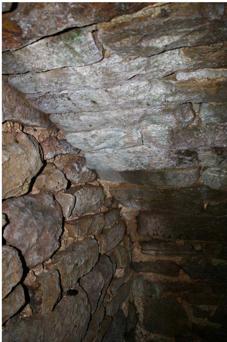
Plate 7: The barrel vaulted roof of the cellar abutting the earlier south gable wall.
