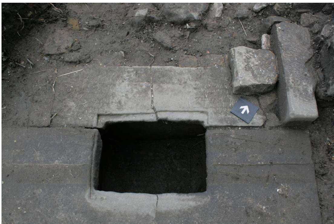
Plate 3: The ash pit and east base of the fireplace surround in the north gable wall, viewed looking north-west.
